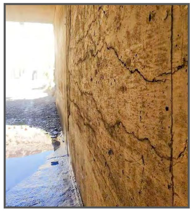
**BULGING AND CRACKING** IN CULVERT WALLS
