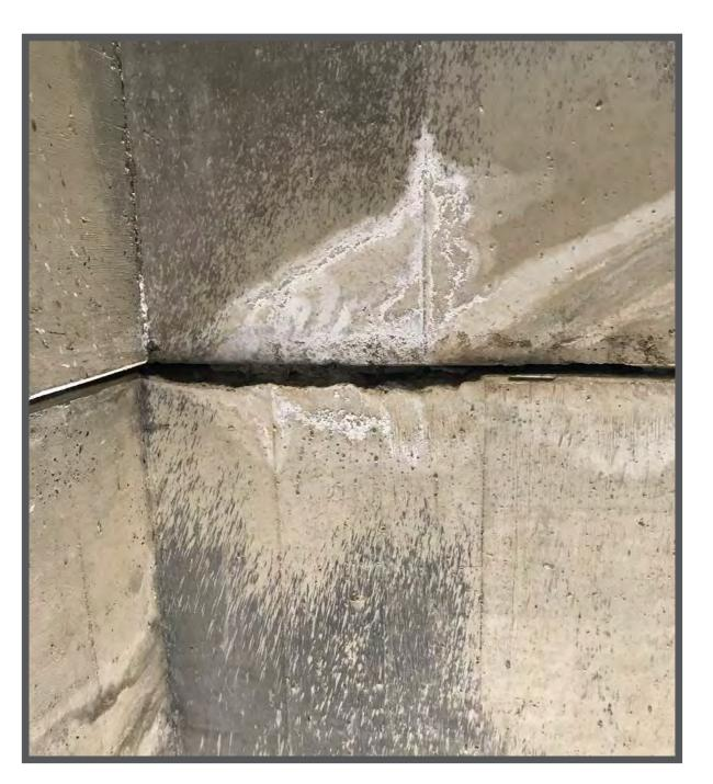
SEPARATION IN CULVERT CEILING
